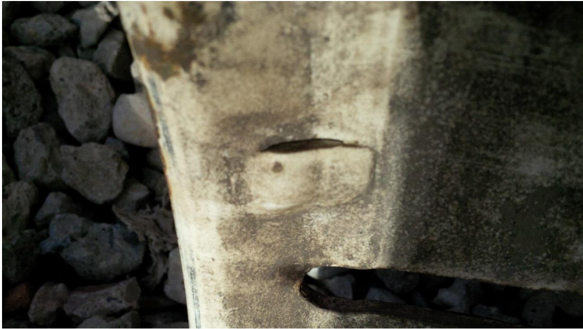
No Damage. Cracks in coating only
